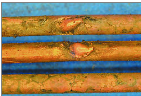
Figure 6.6.5.3.2(e) Mass Transfer in the Form of Molten Material Sprayed from the Arc Location in a Steel Enclosure.
