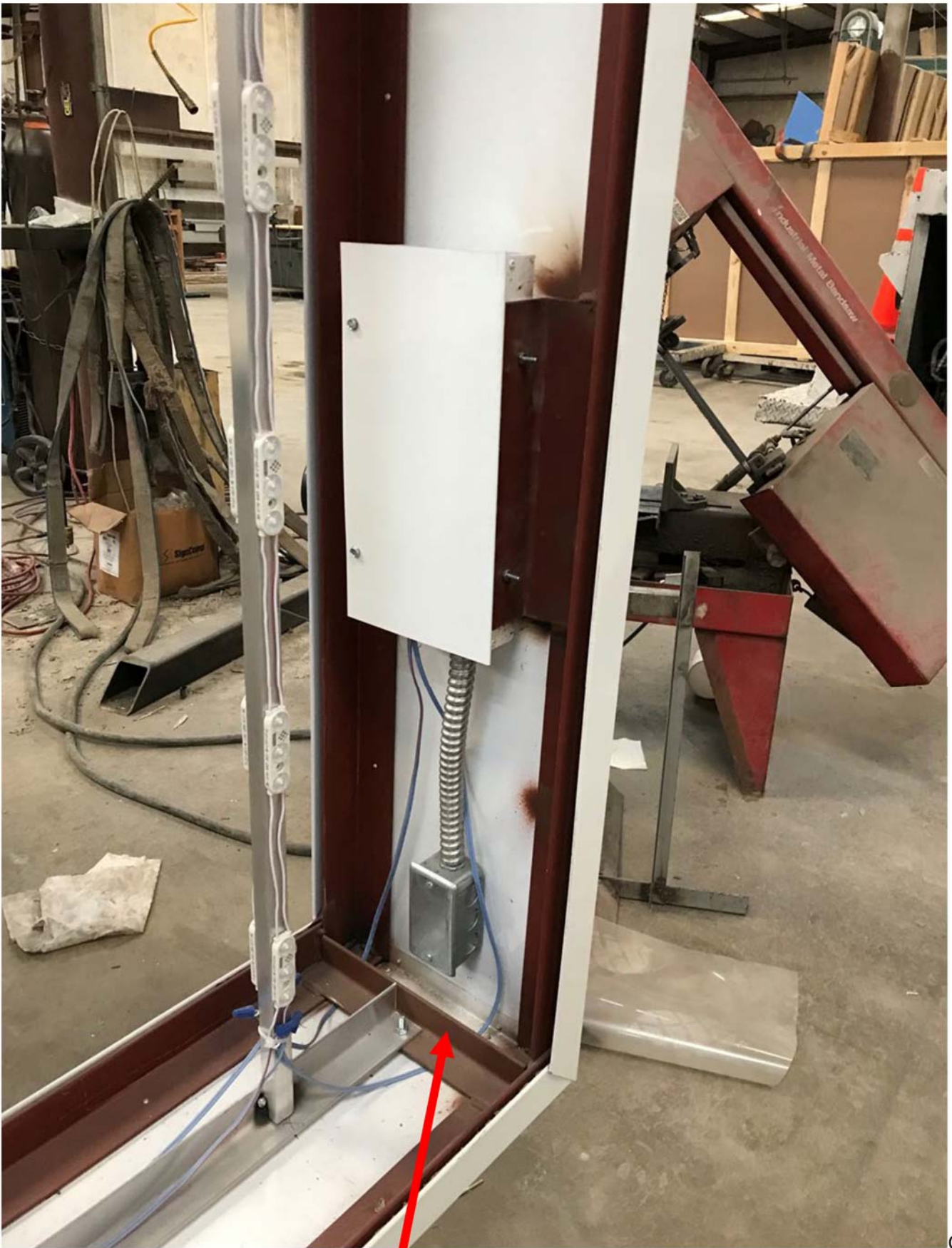
3 wiring method will terminate into a device box.
