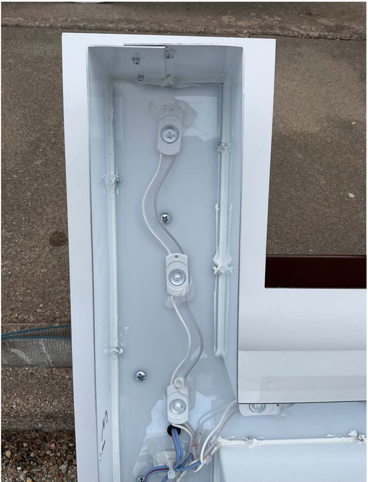
Halo rear illumination with Plexi glass illuminated face. Metal not bonded. 2 wire Class 2 cable installed.
