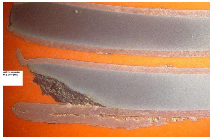
Figure 4b: Corrosion occurred at the ends of the wires. Maximum penetration depth is 0.859 inch.
