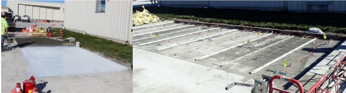
Figure 2. Construction of two ECON HPS test slabs at DSM
