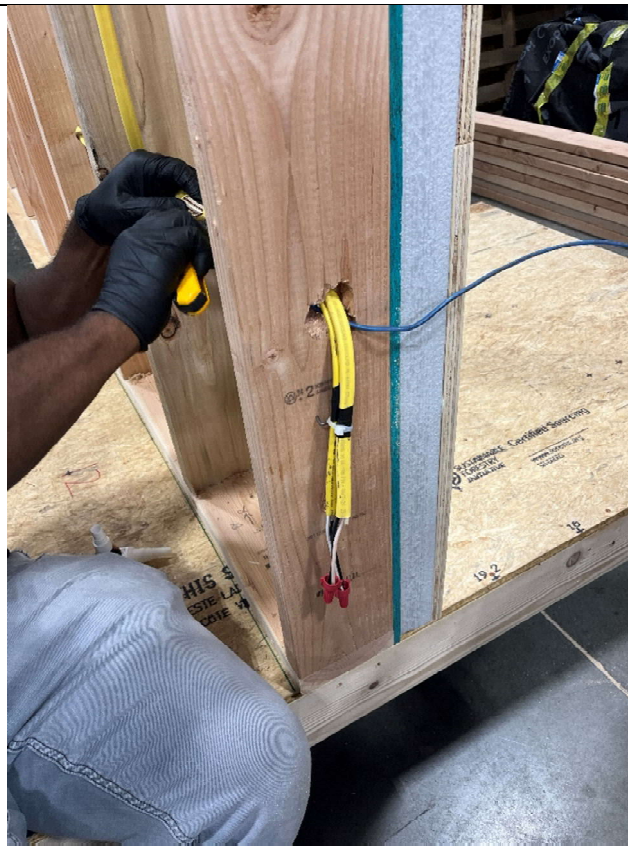
Figure 5 – 10-2 and 12-2 NM-B Conductors Connection at End
