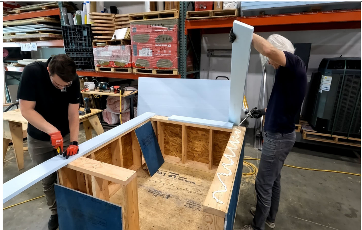
Photo 2 – 2x6 Framing Assembly of Lowest Level
