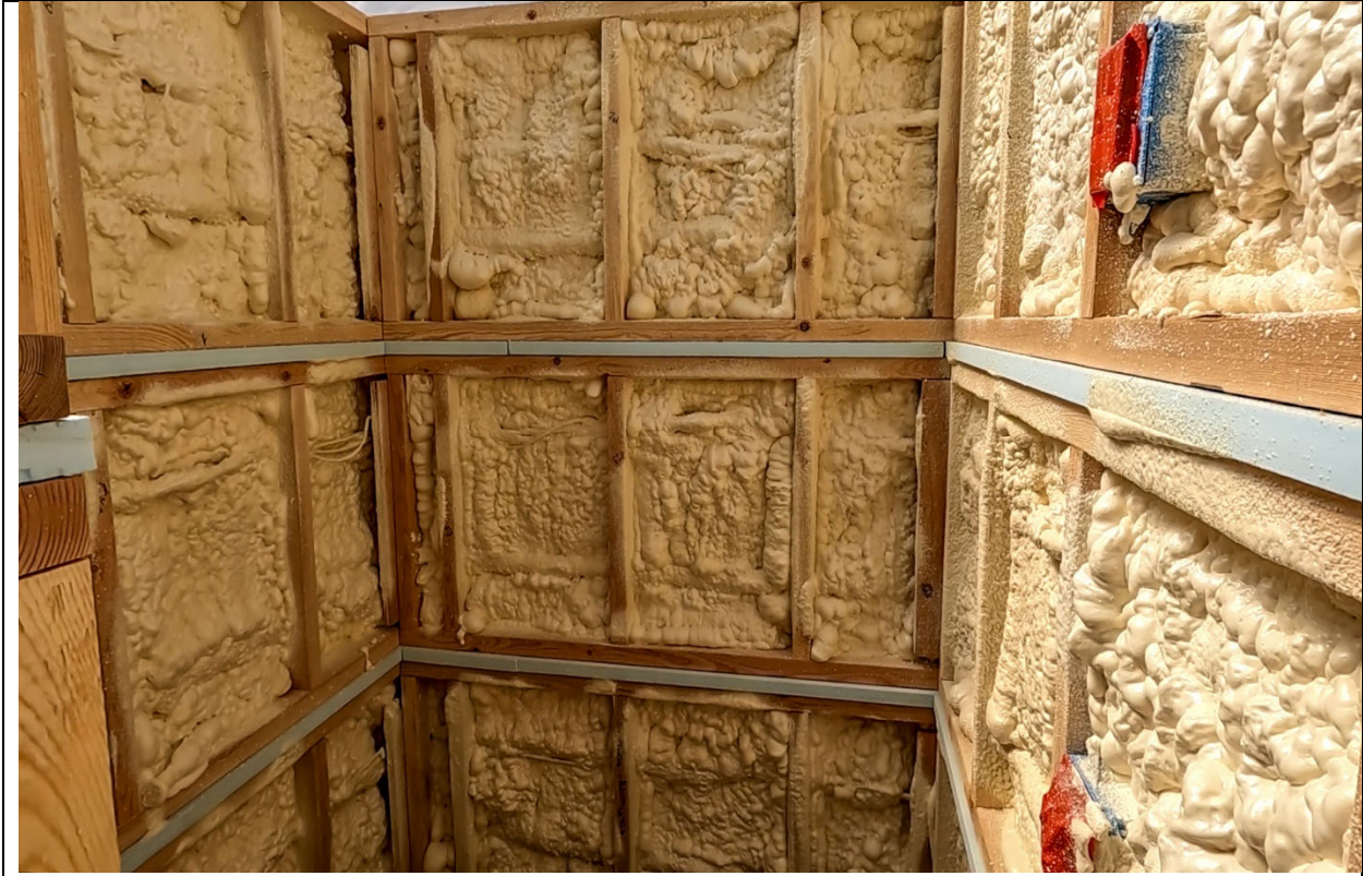
Photo 7 – Test Fixture 2 R30 Spray Foam Insulation
