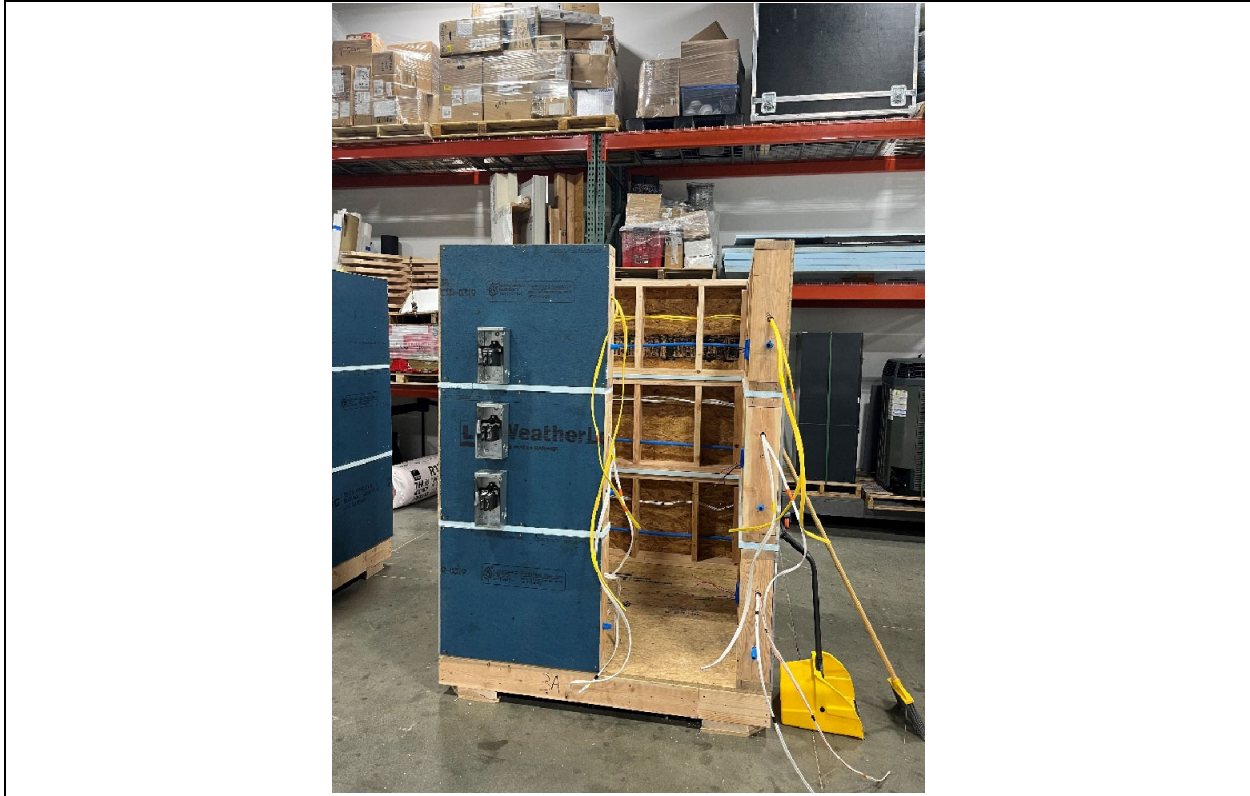
Photo 3 – Wall Test Fixture with Rough Wiring Installed
