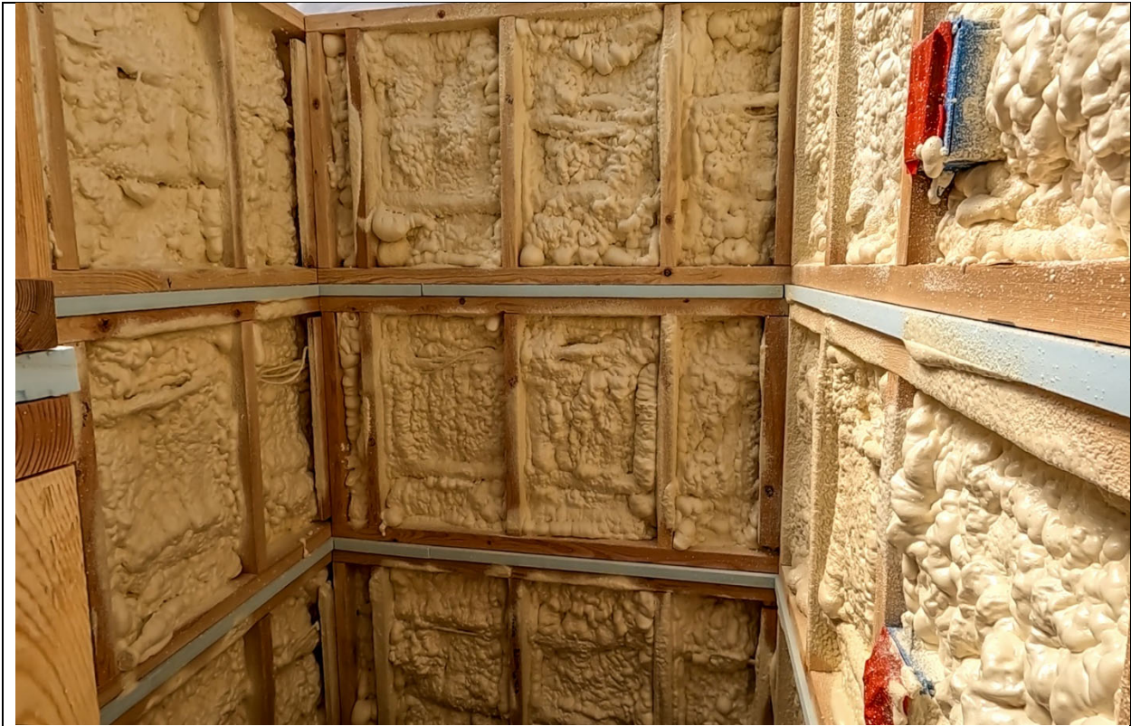
Photo 7 – Test Fixture 2 R30 Spray Foam Insulation
