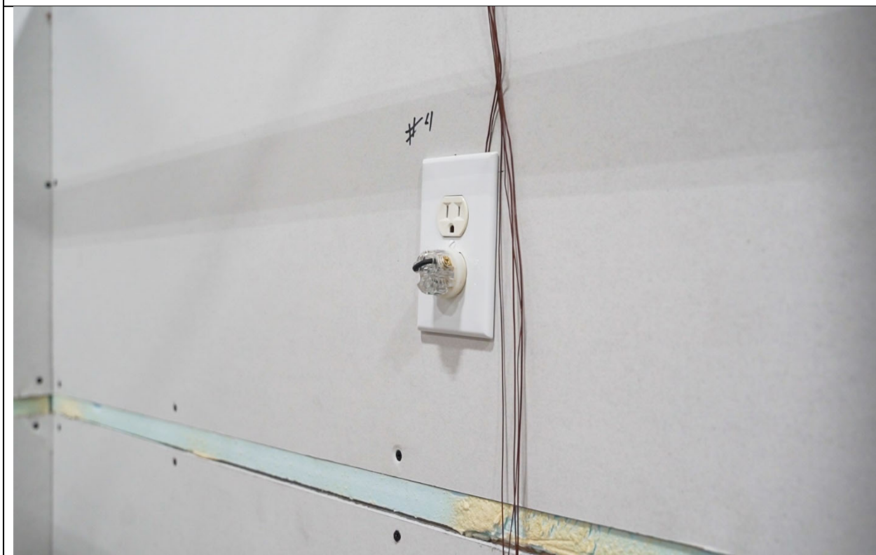
Photo 12 – Receptacle with Thermocouple and Shorting Plug
