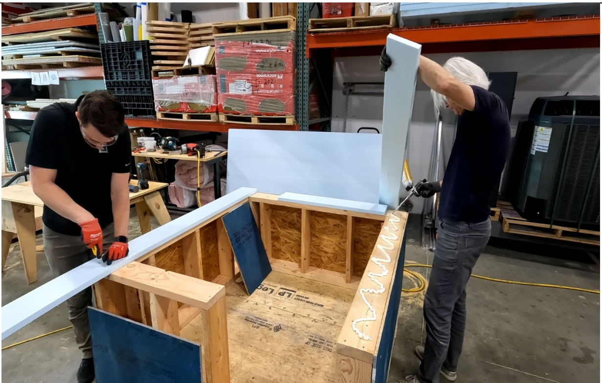
Photo 2 – 2x6 Framing Assembly of Lowest Level
