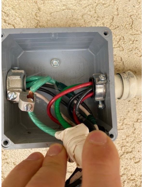
Photo 5 – Non-metallic Junction Box with EMT Raceway
