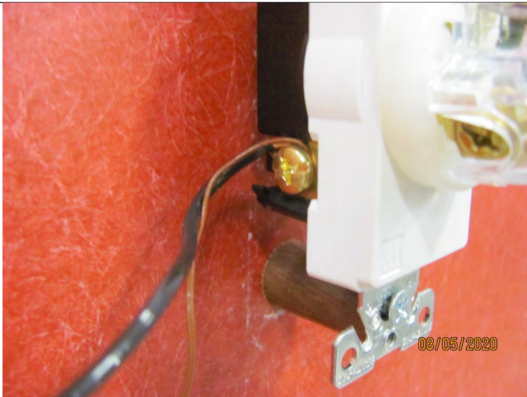
Photo 6 – Typical Installation of Receptacle using Wire Binding Screw
