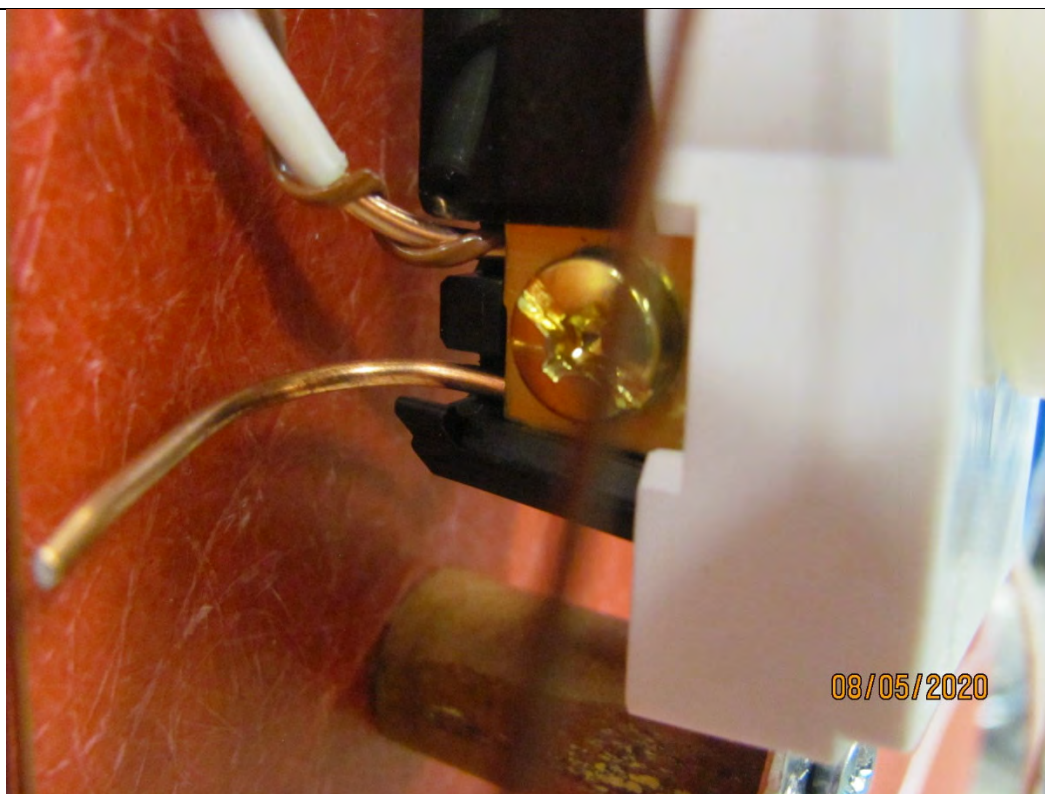
Photo 8 – Typical Installation of Receptacle Two Conductors Back Wired
