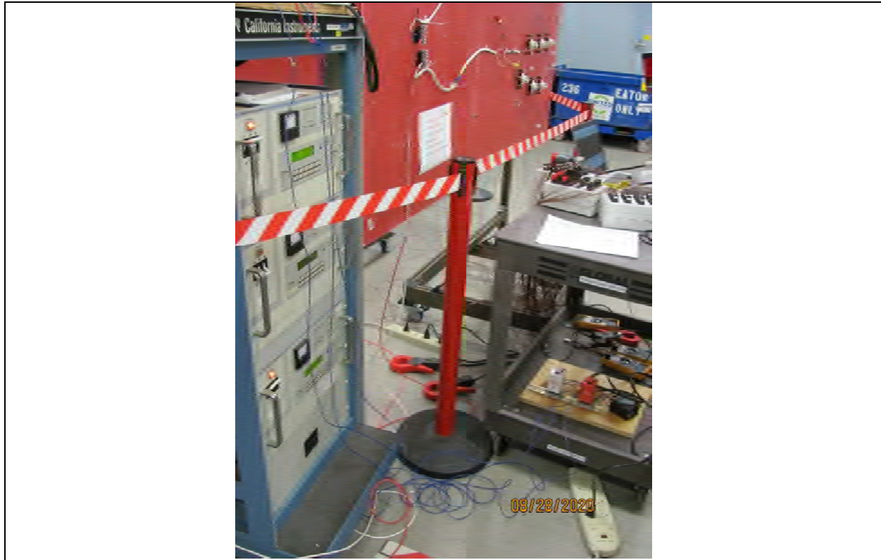
Photo 3 – Power Supply and Datalogger Arrangement
