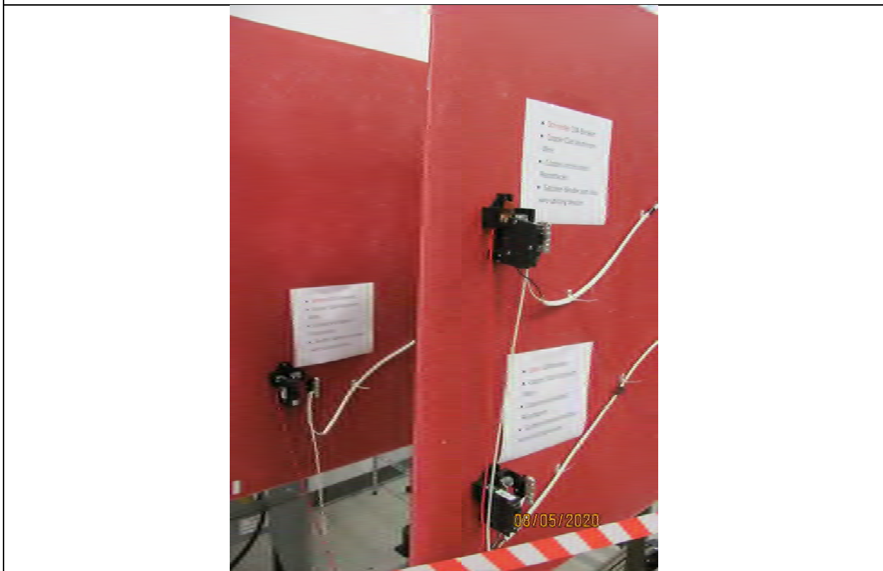
Photo 4 – Copper-Clad Aluminum with Eaton and Hubbell Receptacles
