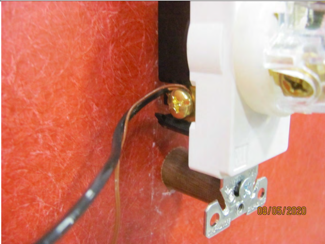
Photo 12 – Typical Installation of Receptacle using Wire Binding Screw
