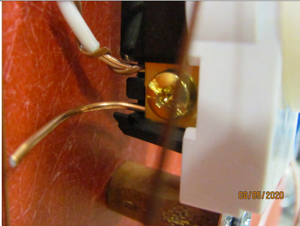
Photo 14 – Typical Installation of Receptacle Two Conductors Back Wired
