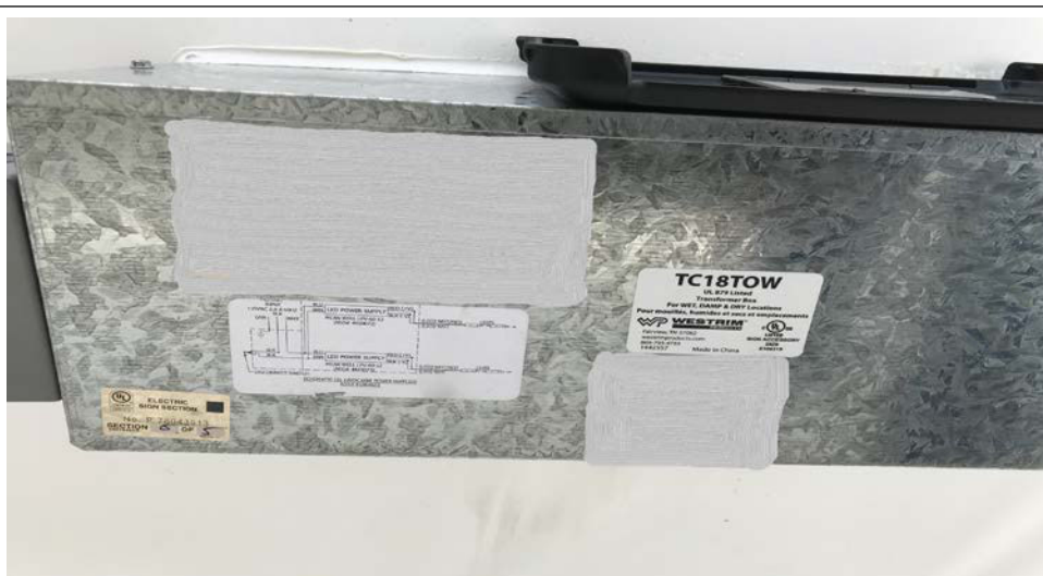
Listed Transformer Enclosure
