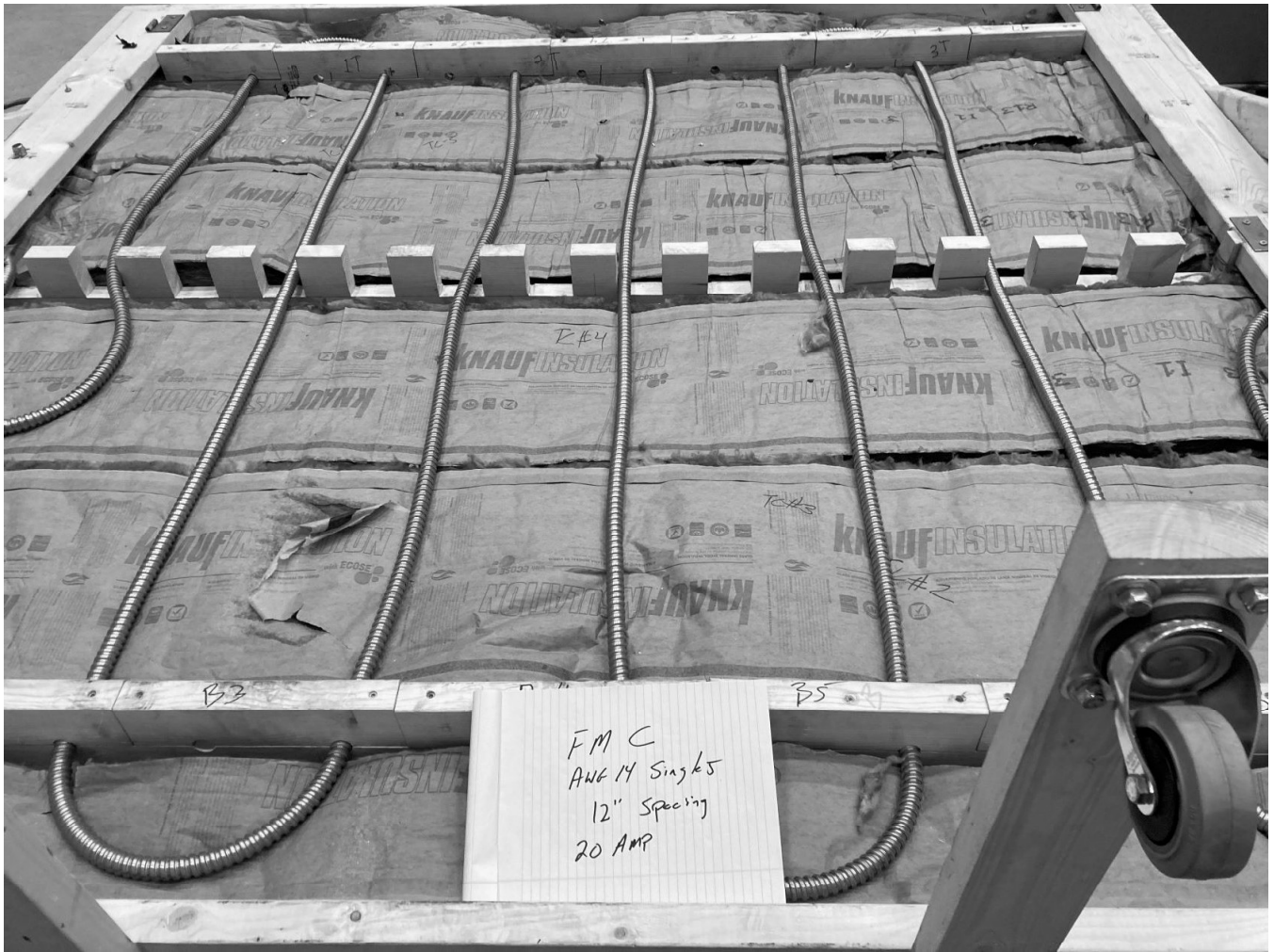
Figure B.6: Flexible Metal Conduit Installed in Apparatus
