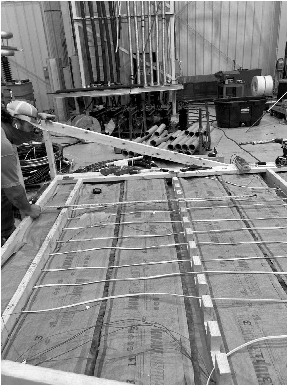
Figure B.9: NM-B Sample Installed in Apparatus in Ceiling Configuration
