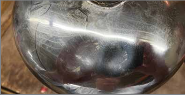
Water extinguisher with dented cylinder.
